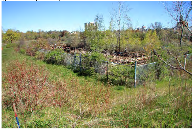
Image 27: North view of oil storage facility remains (API separator).
