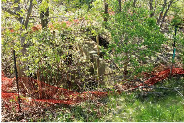
Image 25: South view of oil storage facility remains (phenol separator).
