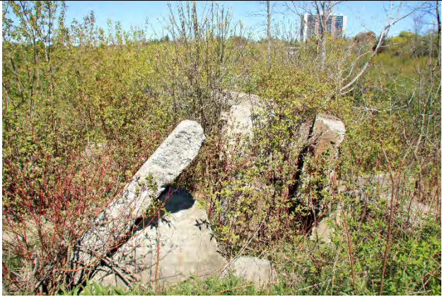
Image 14: Southeast view of poured concrete chunks near former ship channel.
